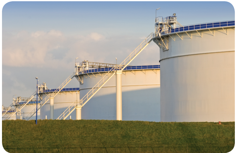
Oil storage tanks.
